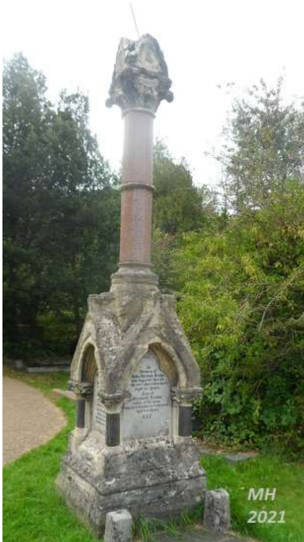
15 Behind the Cloisters [ST 60751 71511] – Arthur Charles Perry d.1952 – Shap Granite from the Lake District showing distinctive domino-shaped crystals of pink feldspar.
