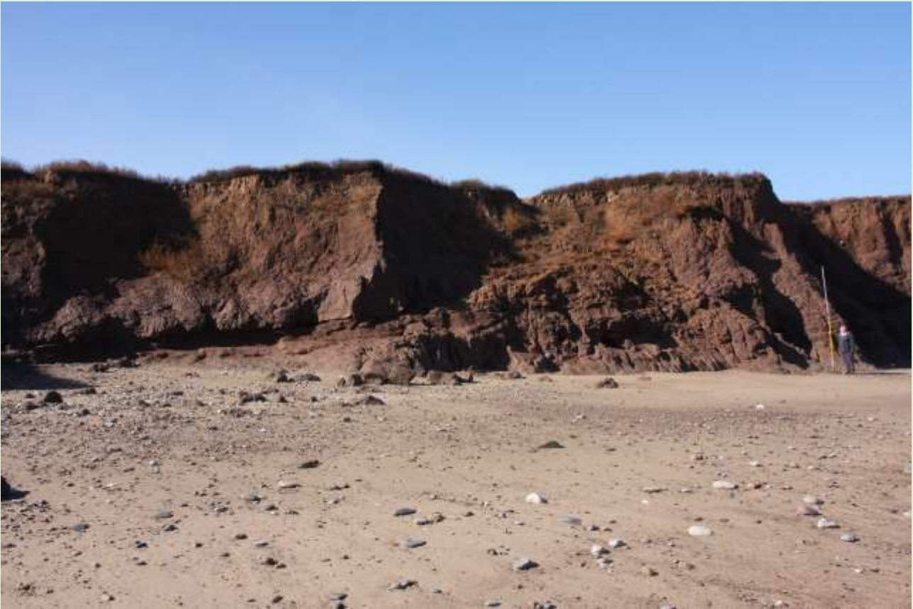
Photograph 1. First pole placement.
